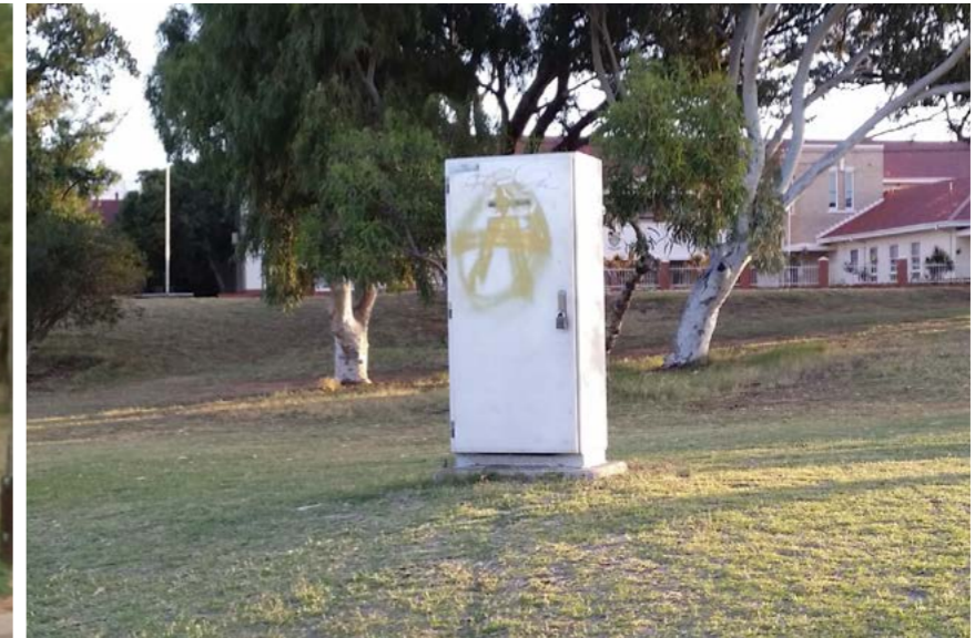
6 EXISTING ELECTRICAL OUTLET
