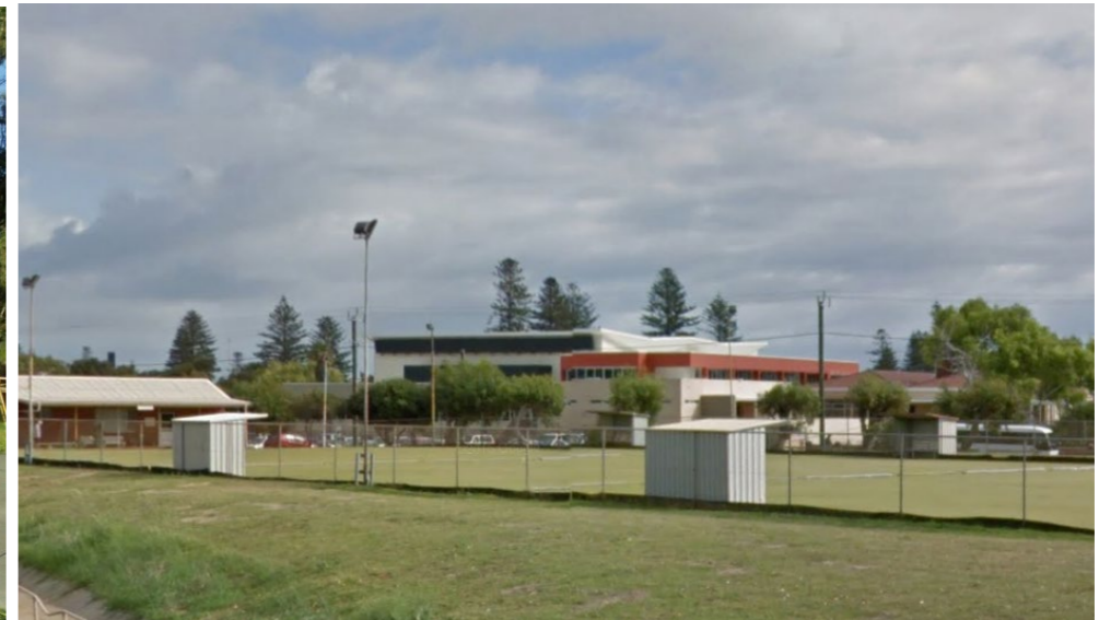
9 EXISTING MAITLAND PARK CROQUET CLUB
