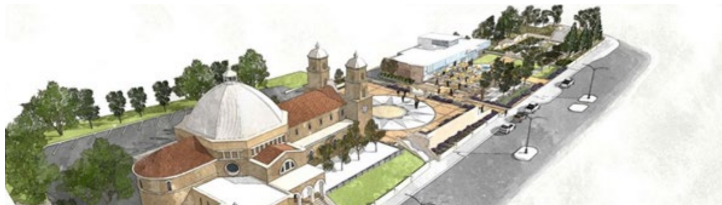
ST FRANCIS XAVIER CATHEDRAL & HAWES HERITAGE CENTRE Source: sfxcathedralproject.com.au
