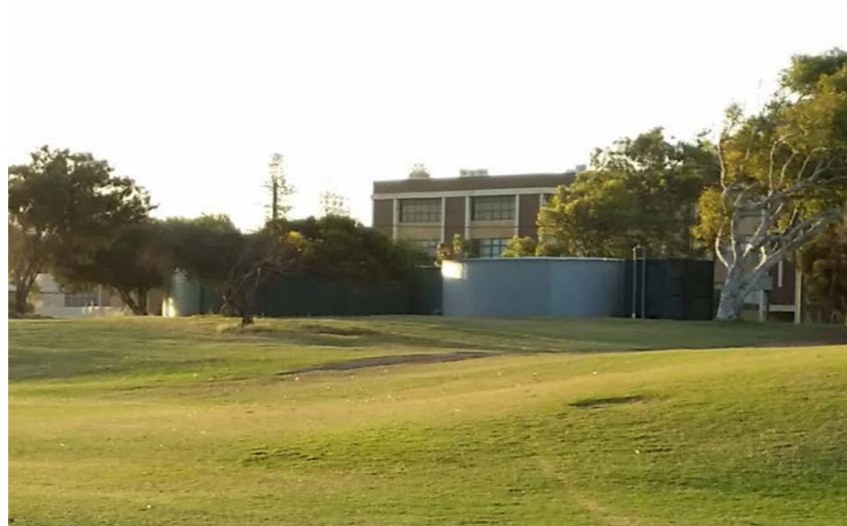
4 EXISTING WATER STORAGE TANKS
